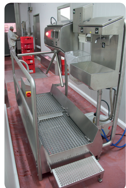
Disinfection basin with drip tray
